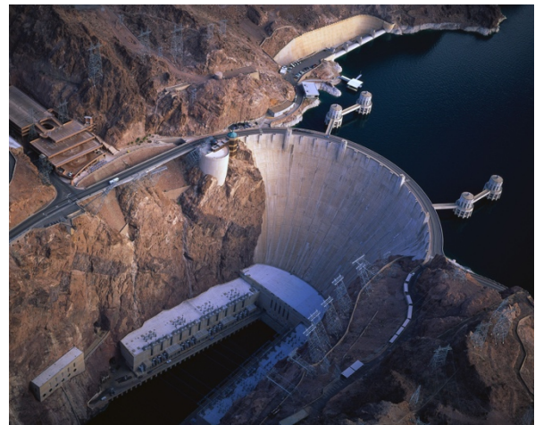
Figure 50. Hoover Dam Hydroelectric Power Plant
