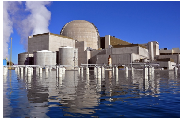
Figure 49. Palo Verde Nuclear Station
