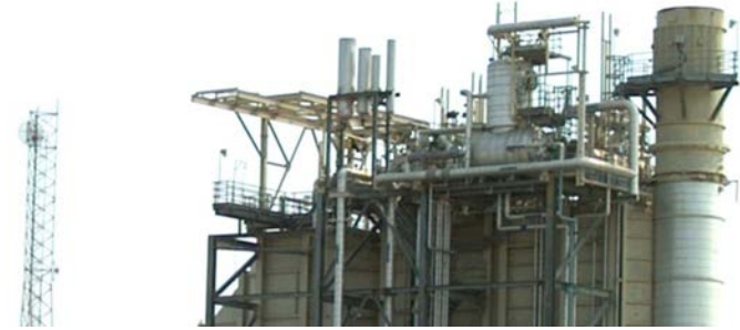
Figure 9. Almond Power Plant
