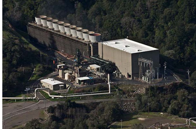
Figure 13. Geysers Geothermal Power Plant
