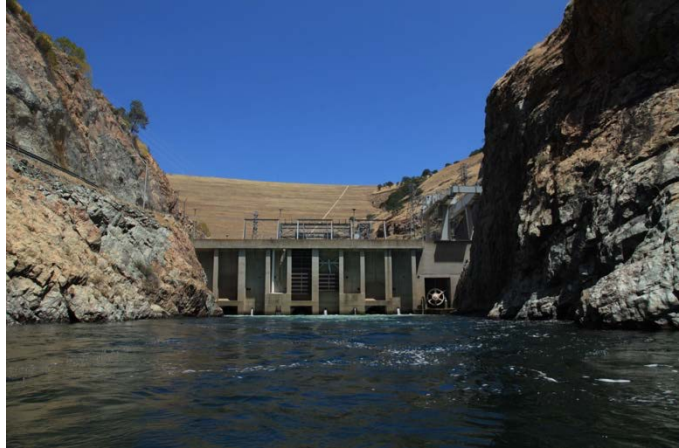
Figure 16. Don Pedro Hydroelectric Power Plant
