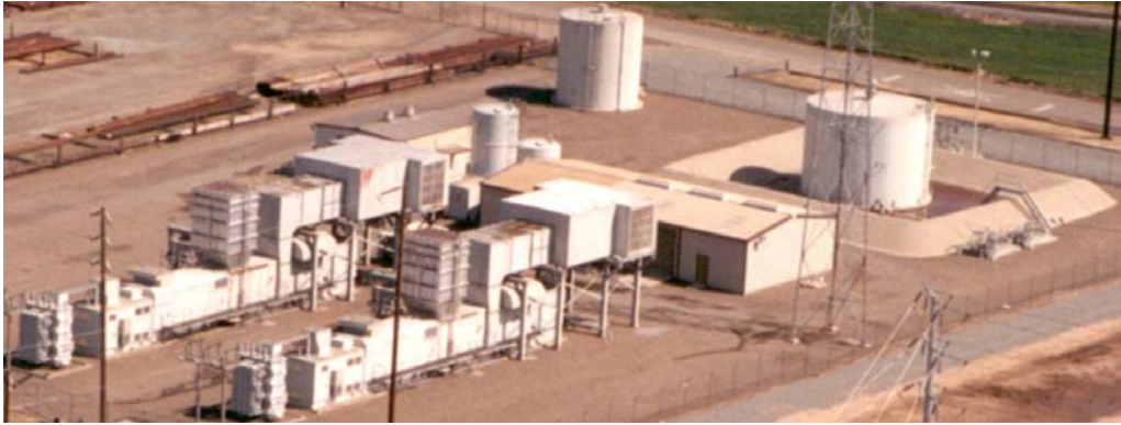
Figure 11. Walnut Power Plant
