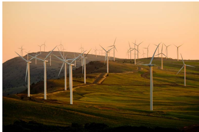
Figure 14. Tuolumne Wind Project Power Plant
